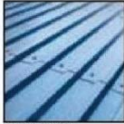
Standing Seam Metal Roof
